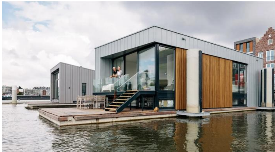
Figure 5. Floating Villa designed by Waterstudio.NL in Dordrecht, the Netherlands
